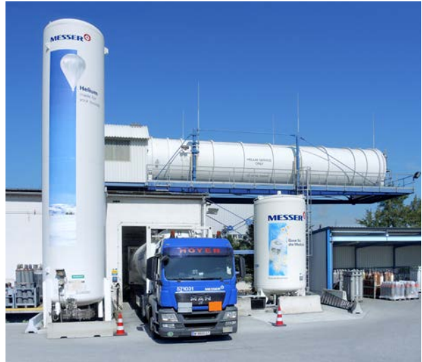
120,000 l horizontal tank container for liquid helium
